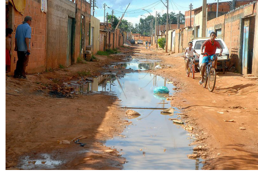
An open sewer in a Brazilian favela.
